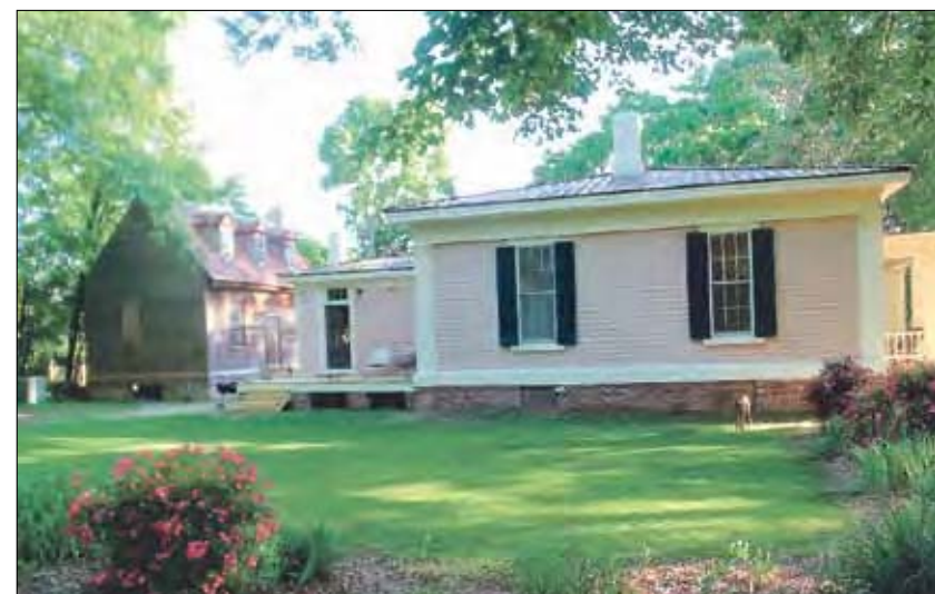
The 800-square-foot, 1790 structure behind the home, moved from another property, was a “law academy” used for teaching law students.
